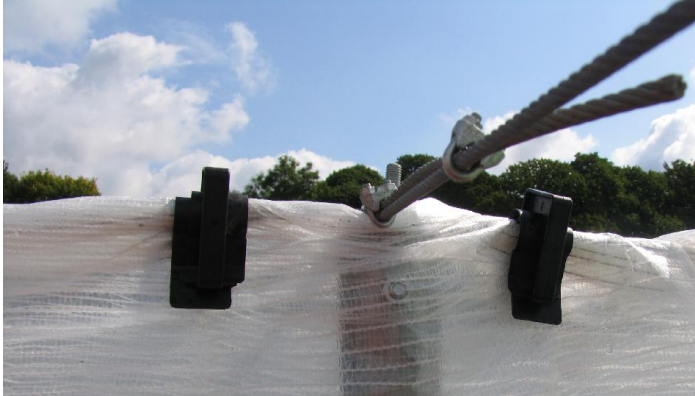
Picture 2: Fix a clip on both sides of the pole. The two clips are closed in direction of the pole.
